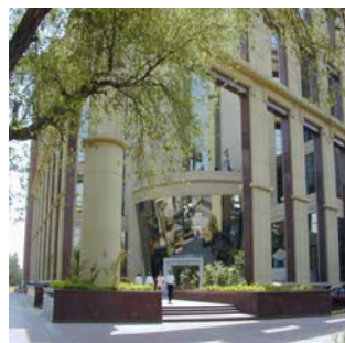
Picture of Hero/ITES Contact Center/ BPO facility near New Delhi
